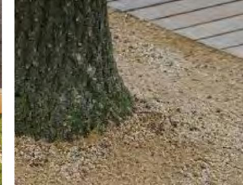
Figure 195. Consolidated/self-binding gravel to tree pits
