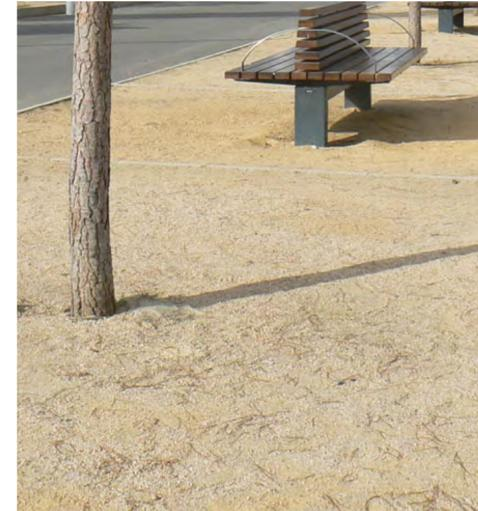
Figure 189. Consolidated/self-binding gravel
