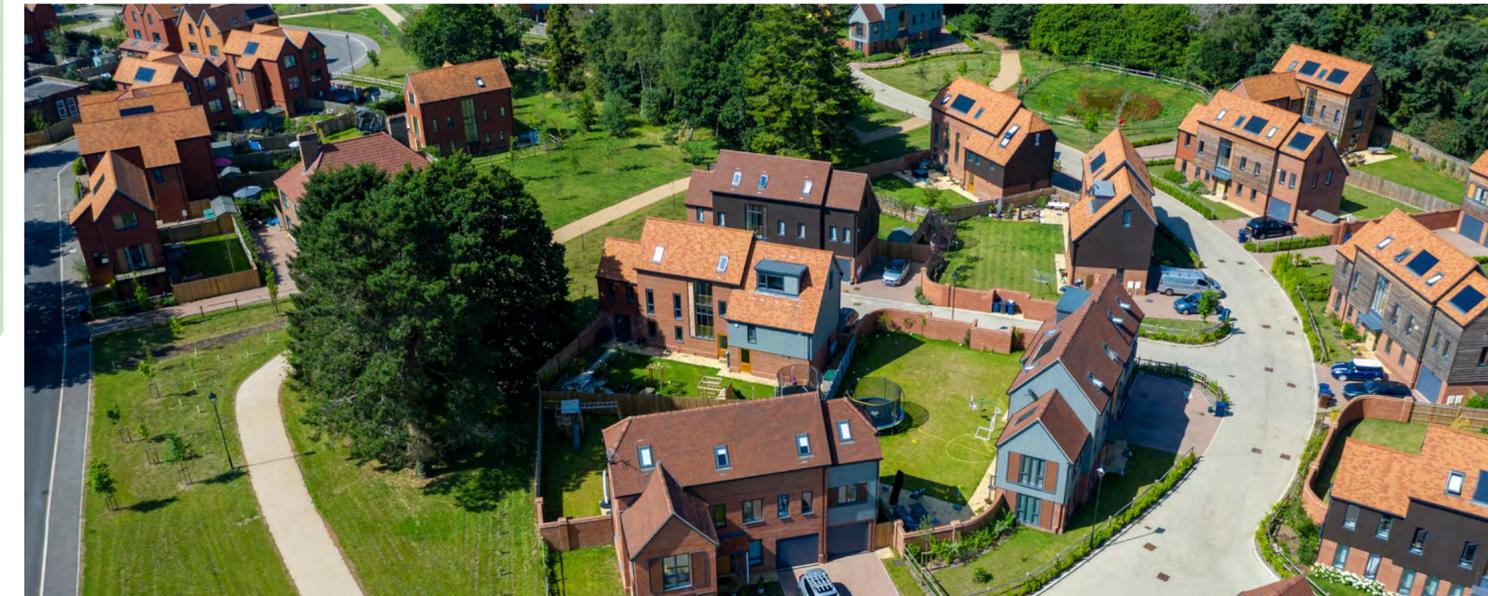
Figure 222. Roofs of adjacent buildings (even when varying in shape) must be designed together so they form a composition in terms of their type, scale, pitch, orientation and projecting elements. Leithfield Park, Surrey - HTA Design
