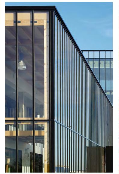
Figure 131. Emphasis on verticality with the use of curtain walls. Alconbury Incubator - AHMM Architects
