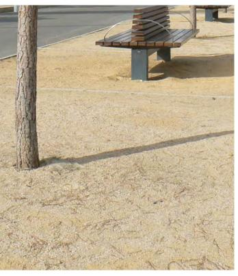
Figure 189. Consolidated/self-binding gravel
