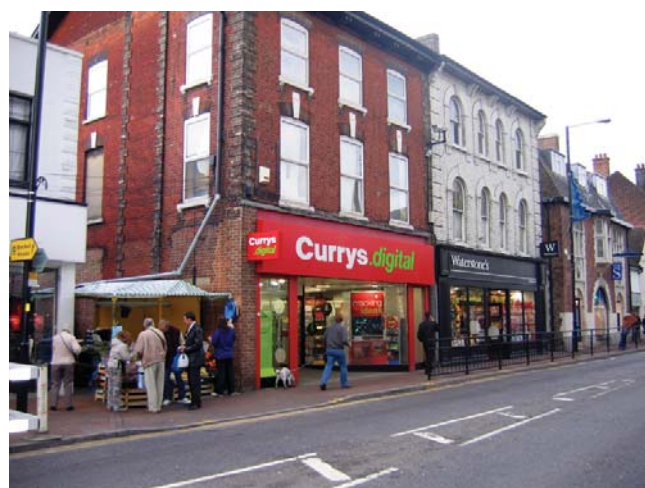
Currys Digital: Again the common problem of a too deep fascia designed to shout out for custom rather than compete with the more subtly designed shopfronts. There is nothing traditional about this shopfront and it has been designed for the maximum impact on the High Street. The deep entrance has been designed to increase window displays but distracts only further from the High Street.
