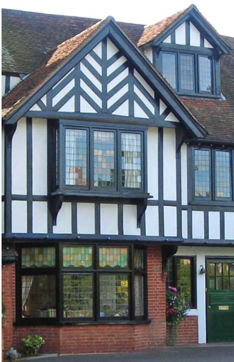
Fig. 15 False half timbering, Ardtully.
