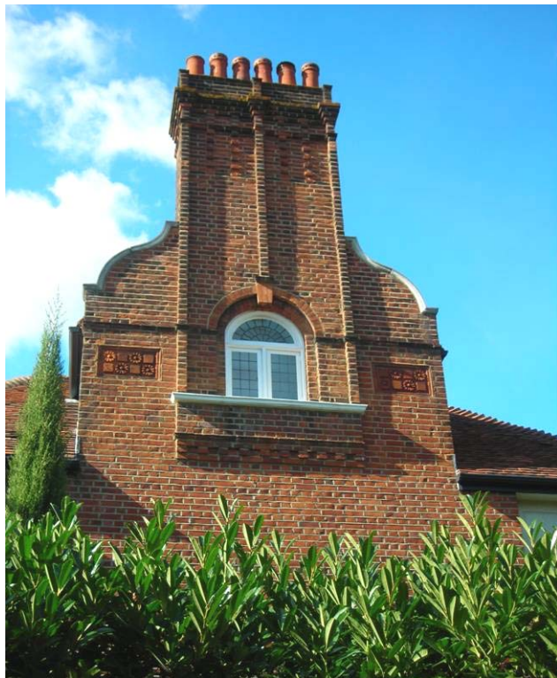
Fig. 16 English bond brickwork, The Gate House.
